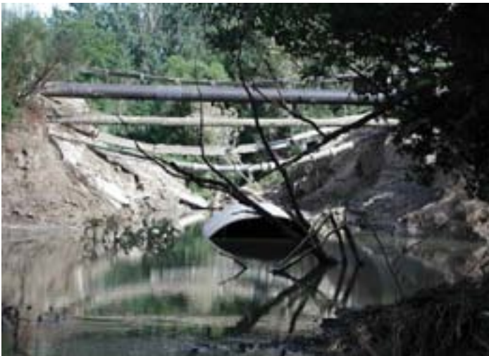
Culvert on Toronto's Finch Avenue at Black Creek Destroyed by August 19, 2005 Storm
